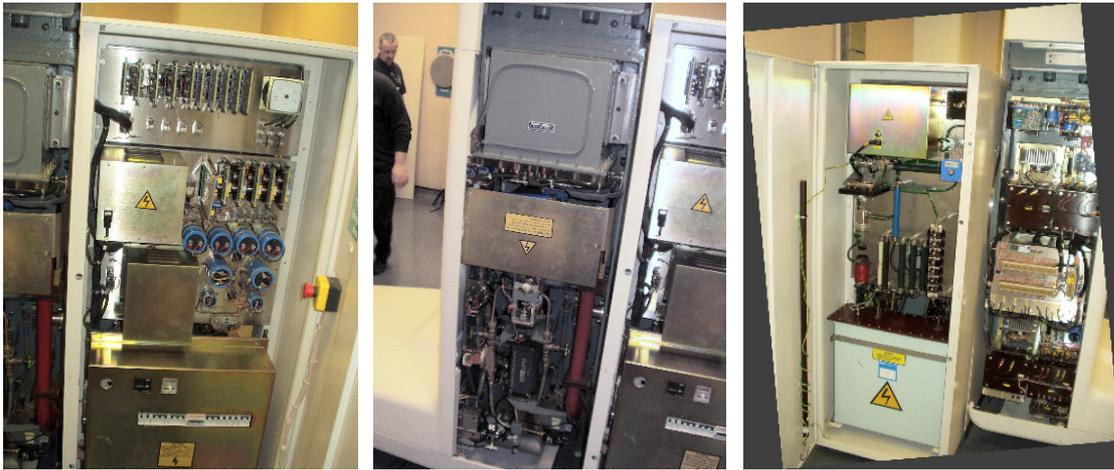
The accelerator power circuits (left), the pulsing circuits (middle) and the modulator and focus supplies (right). John Draper is in the background of the middle image, wandering, along with everyone else, how not to get roped in to this project.
